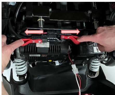
Figure 9: Disconnecting the batteries.
